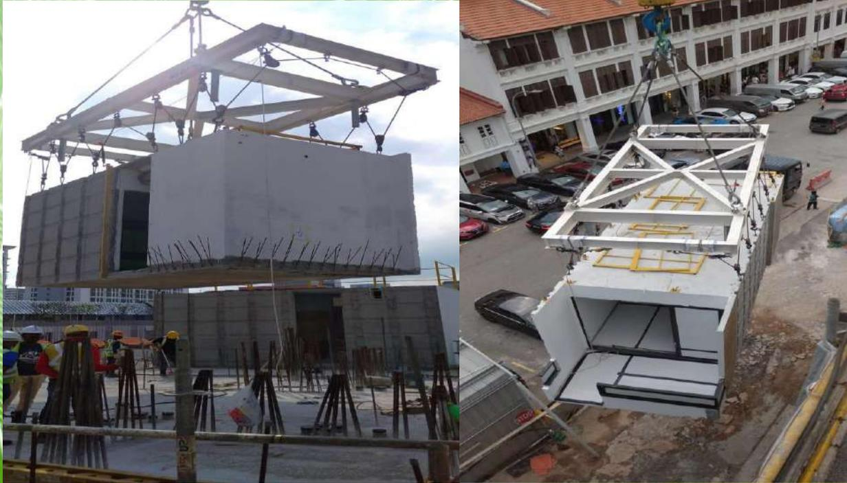
Prefabricated Prefinished Volumetric Construction (PPVC)
