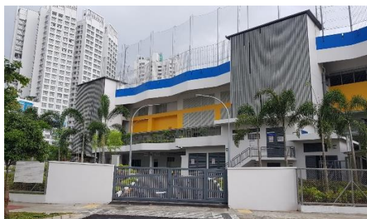
Primary School @ Punggol Way (Punggol Site 26) Client: Ministry of Education Approx Contract Value: S$49.9 million
