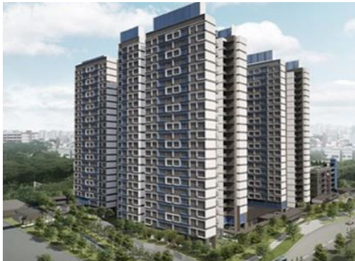
Kallang Whampoa C43 Client: Kienta Engineering Construction Approx Contract Value: S$10.4 million
