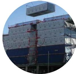
PREFABRICATED PREFINISHED VOLUMETRIC CONSTRUCTION (PPVC)
