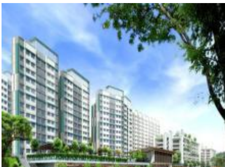
Woodlands C29 & C30 Client: Housing Development Board Approx Contract Value: S$204.5 mil
