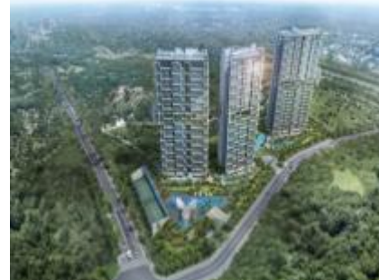
Eco Sanctuary Client: SP Setia International Approx Contract Value: S$135.4mil
