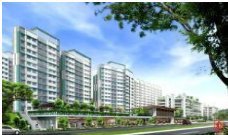
Woodlands N7 & C30 Client: Housing Development Board Approx Contract Value: S$204.5 mil
