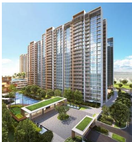
Sol Acres Executive Condominium Client: MCL Land Pte Ltd Approx Contract Value: S$276.0 million TOP in 1Q2018
