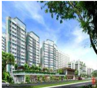
Woodlands C29 & C30 Client: Housing Development Board Approx Contract Value: S$204.5 mil
