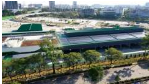
Ulu Pandan Bus Depot Client: Land Transport Authority Approx Contract Value: S$69.9 mil
