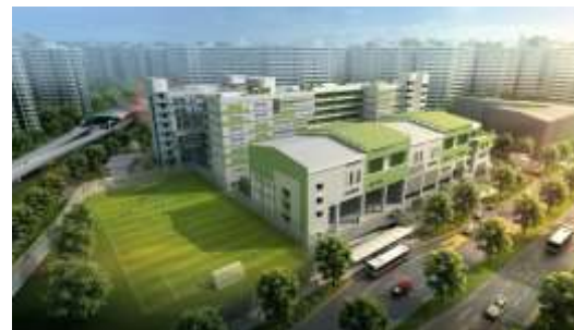
Primary School along Punggol Central / Punggol Way Client: Ministry of Education Approx Contract Value: S$53.9 million
