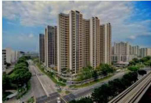
Executive Condominium Sol Acres Client: MCL Land (Brighton) Pte Ltd Approx Contract Value: S$276.0 mil
