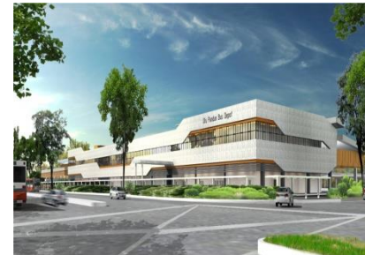
Ulu Pandan Bus Depot Client: Land Transport Authority Approx Contract Value: S$69.9 mil
