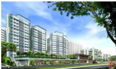
Woodlands C29 & C30 Client: Housing Development Board Approx Contract Value: S$204.5 mil
