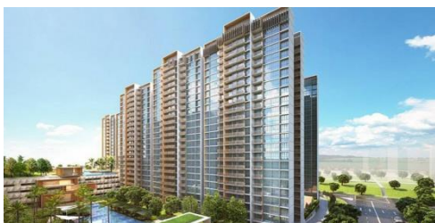
Executive Condominium at Choa Chu Kang Grove Client: MCL Land Pte Ltd Approx Contract Value: S$276.0 mil
